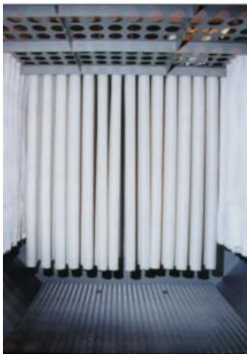
Figure 8. Inside Of Baghouse
