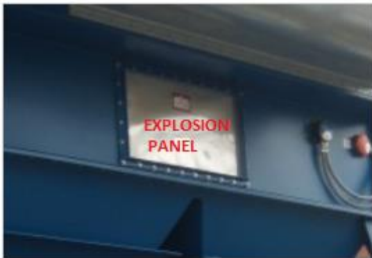
Figure 27. Explosion Panel
